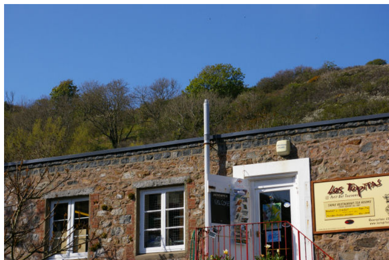
Figure 4 – Antenna at Petit Bot site is disguised as a PVC pipe
