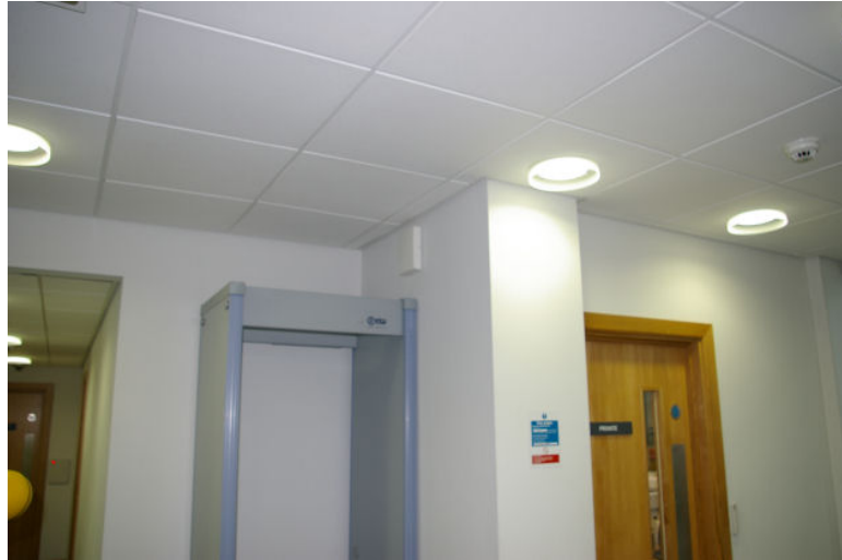
Figure 8 - Antennas at the Court House's main hall
