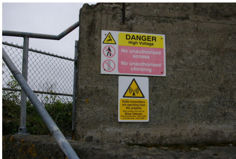
Figure 11 - Typical C&W RF hazard sign
