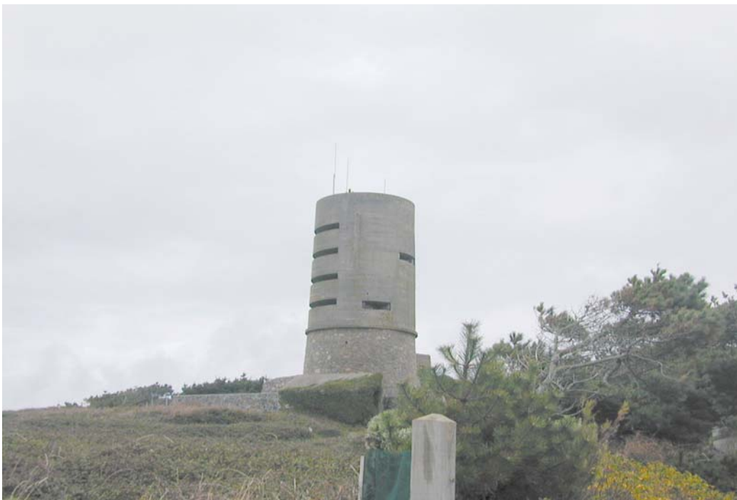
Roof Top Mounted
